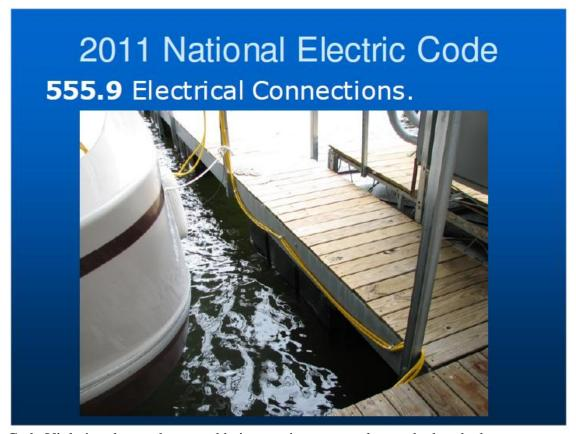
Code Violation due to shore cord being semi-permanently attached to dock.
